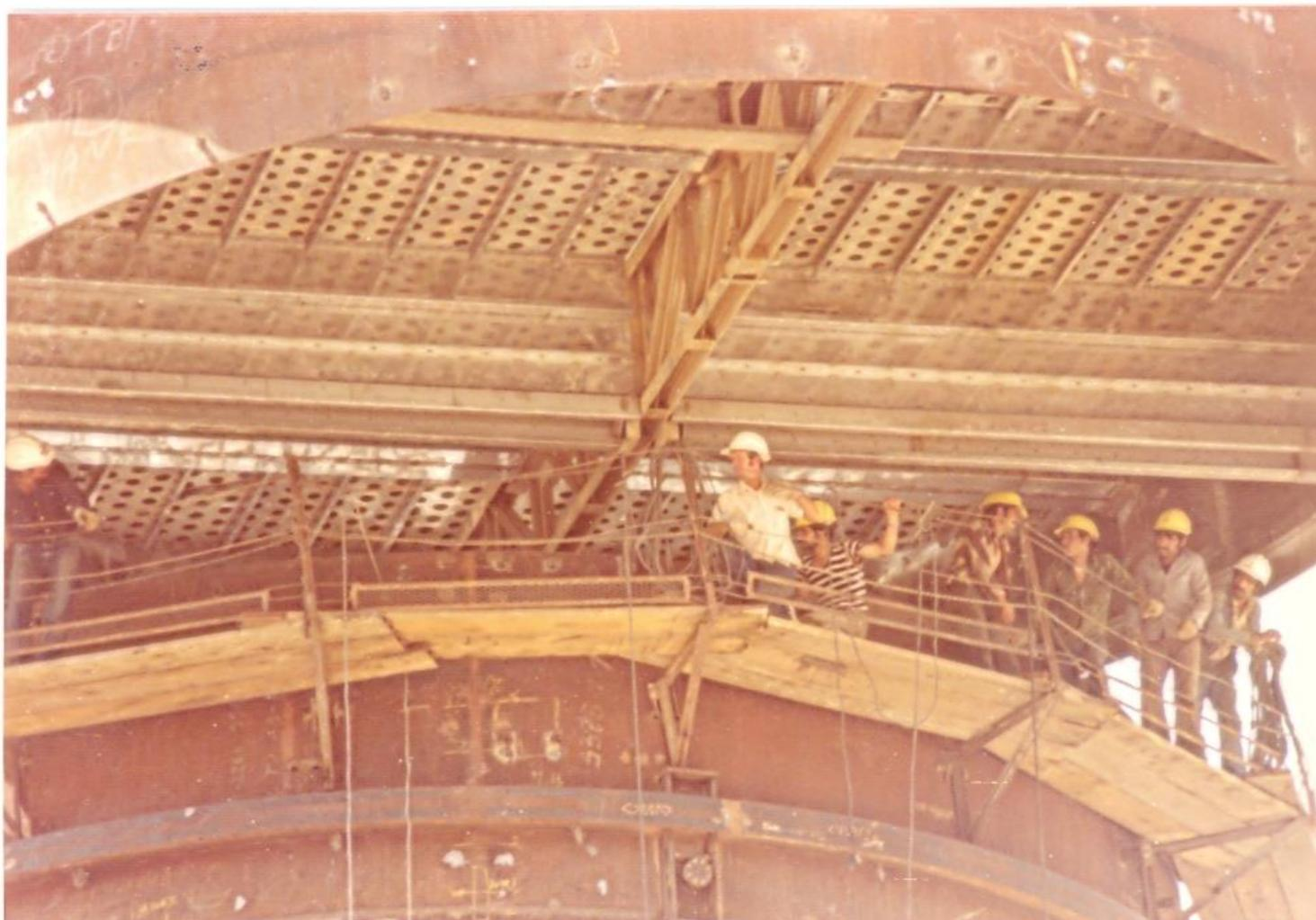
The photo below shows the section landed on top of the existing sections and is ready to be fitted up. The two sections that must be welded together can always be expected to be out of round with each other, Murphy will
