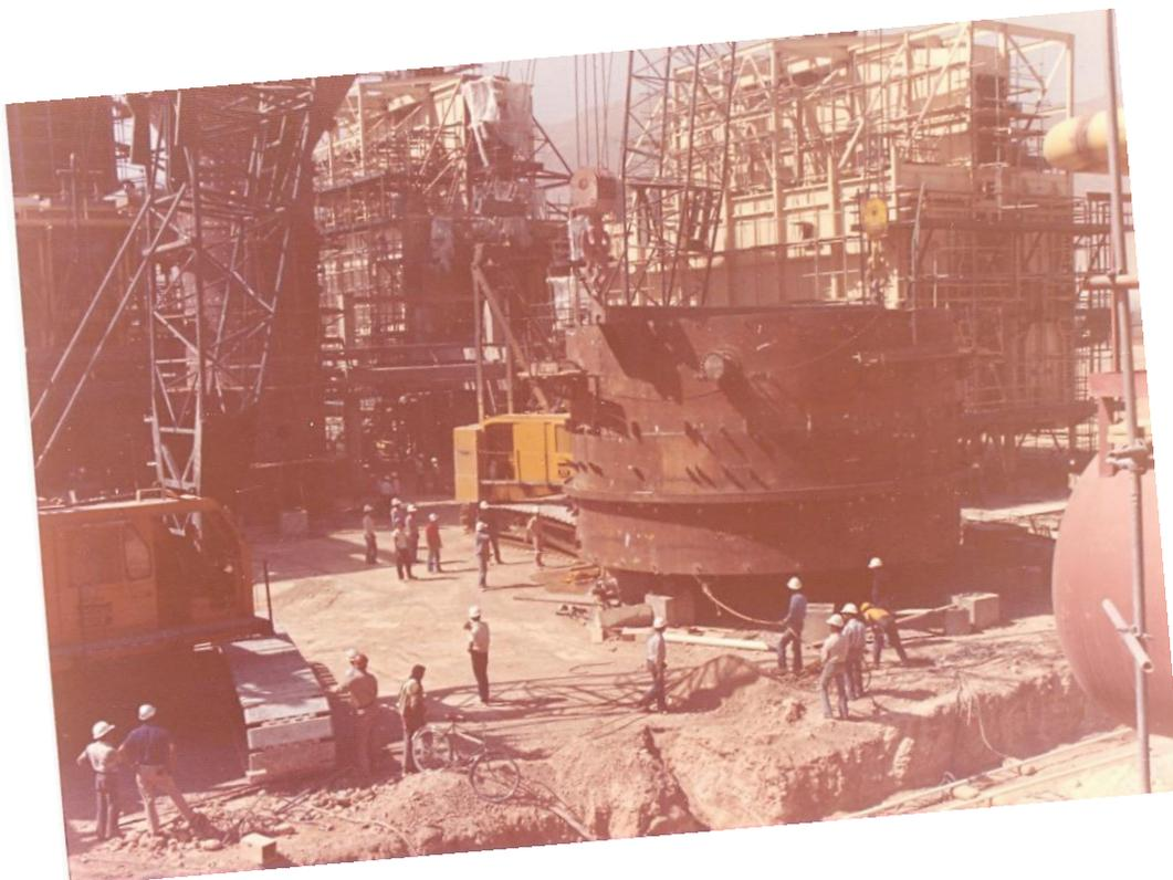
The photo below shows the section being swung between the cranes so it will be in a position in front of the cranes to be walked forward, hoisted and set on the sections that are already set.
